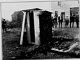
Thirty Minutes After Starting Fire
